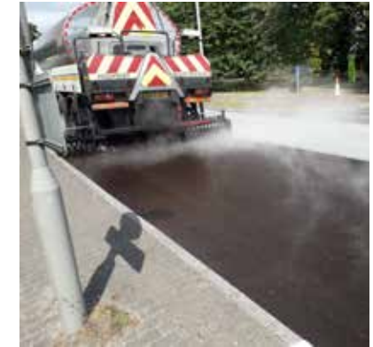
Road investment – highway maintenance in BCP.
